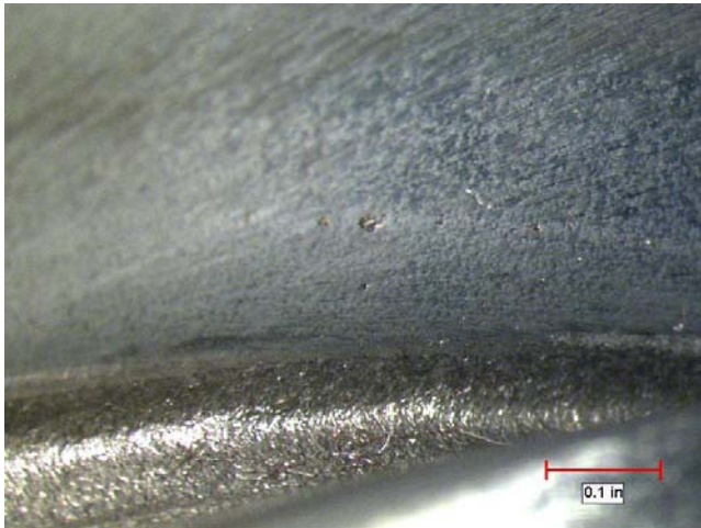
FIGURE 10: AREA OF LOCALIZED HIGH CONTACT STRESS AT THE BOTTOM OF CONTACT WITH LINE OF PITTING AT THE TOP.
