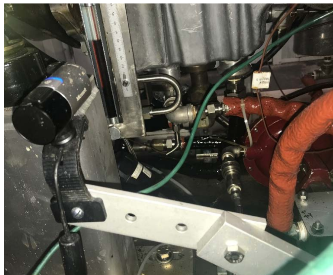
FIG A11.3 Camera Used to View Oil Pan Sight Glass and Scale
