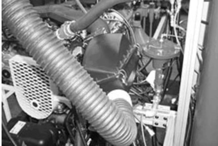
FIG. A7.21 Intake Air Supply System, Air Cleaner, Resonator and Idle Load Control (Replace)
