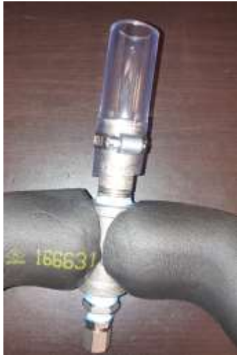
Fig. A8.16 Installing the top hose
