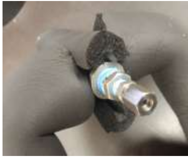
Fig. A8.18 shows sliding the insulation over the top hose
