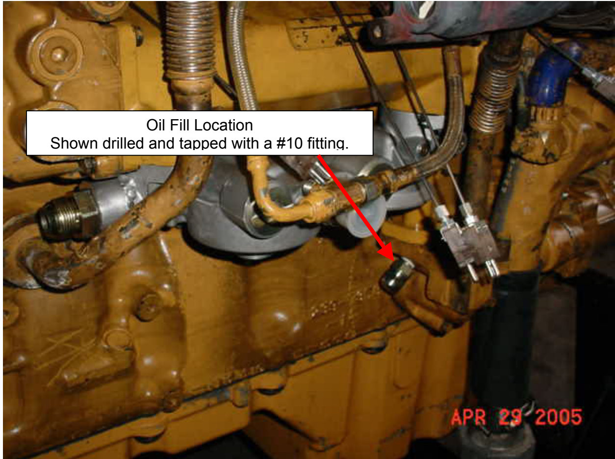
Fig. A4.21 Pressurized Oil Fill Location
